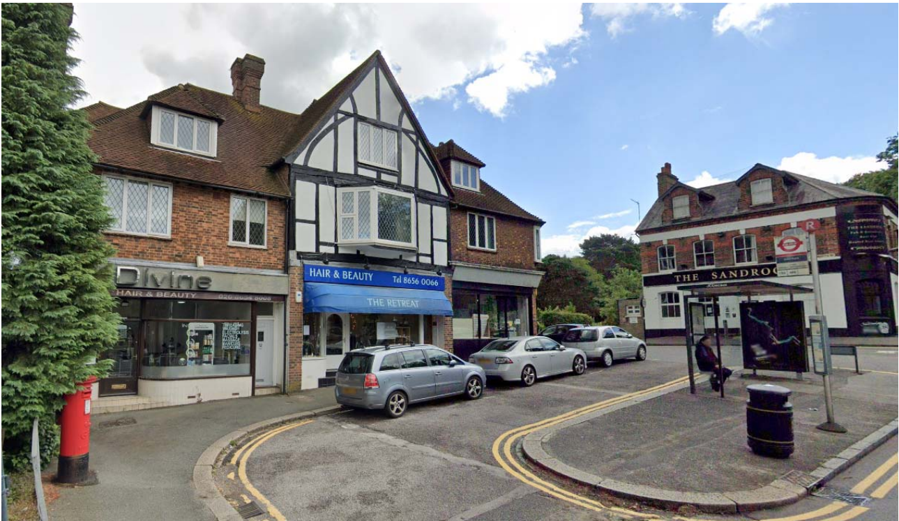
Figure 4: The Sandrock (right) and Adjacent Dominant Building
